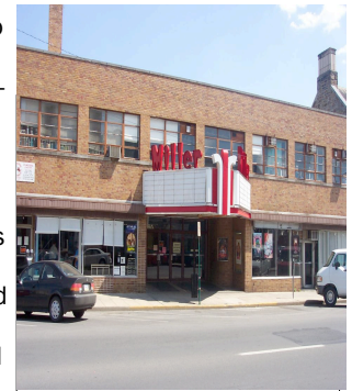
Miller Theatre marquee rehabilitation
