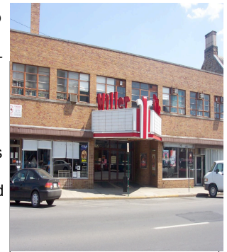
Miller Theatre marquee rehabilitation
