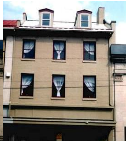
Former Bank Annex after rehabilitation Now offices of Sun Home Health Services
