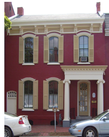
Clear Concepts Office after rehabilitation utilizing Design Challenge Grant funding
